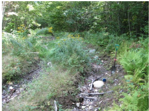
Soil Disturbance Class (SDC) 3: Gully erosion, bare soil, and rutting greater than one foot deep in a skid road.
